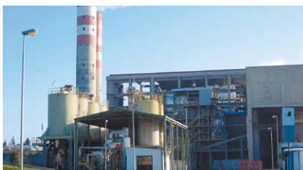
Waste Incineration Plant
